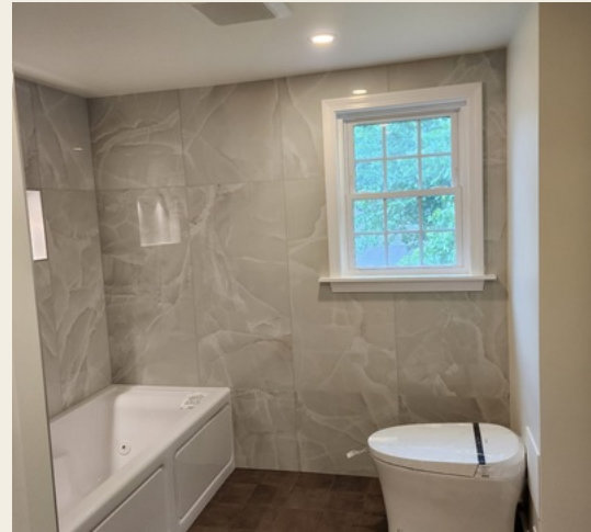
Bathroom tile and finishing
